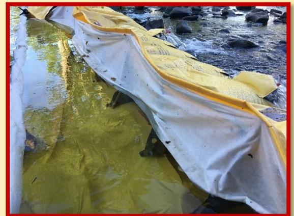
**Optional measure:** Inserting a small number of dowels or poles in the inner walls will **prop the dam open** and limit the assistance requirements. This configuration also assist in fixing filter clothes or sorbent booms. Convenient on dry ground / ditch to protect from potential spill release confinement.
