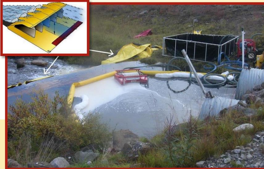
The instant dams, deployed perpendicular to a stream or ditch, create optimum quiet, deep water response zones out of small or large, slow or swift running streams. Cleaning equipment such as sorbents, booms, skimmers or vacuum units can be used efficiently, even in what was initially a few inches of water. The **Water-Gate** system is adapted for emergency response on roads, in ditches, streams, or any other location where it can be deployed.
